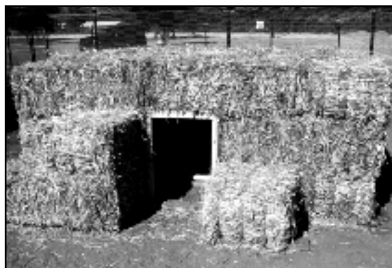
Simple straw house, 4x6 foot interior, 10 x10 foot rooftop play area, and steps!
